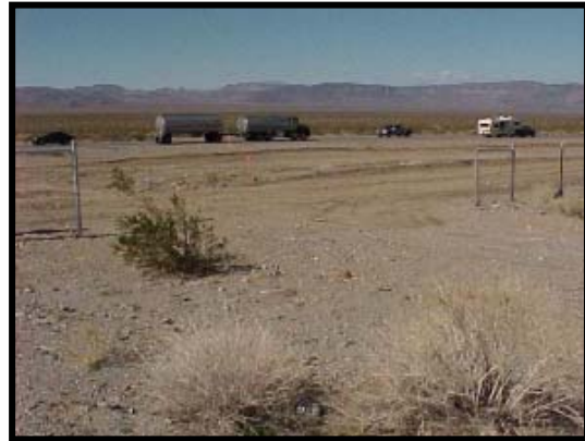
Cattleguard needed at US95 – mile marker 37
