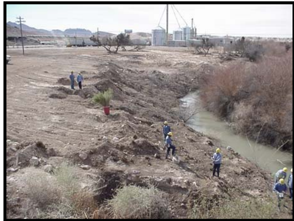
One Side Cleared With Restoration In Progress
